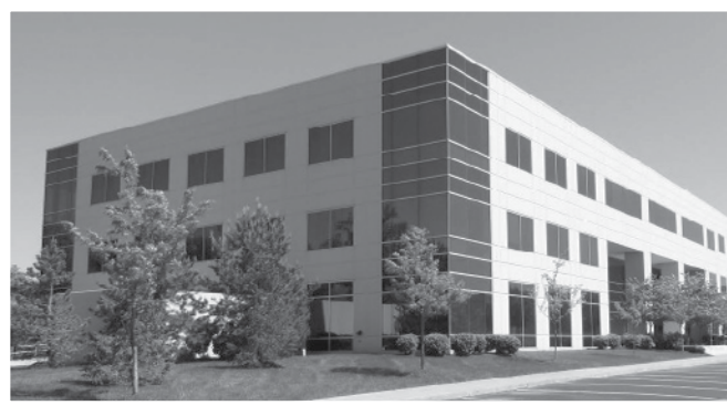
New Headquarters Building 2016-Present 36 Research Park Court Weldon Spring, Missouri
